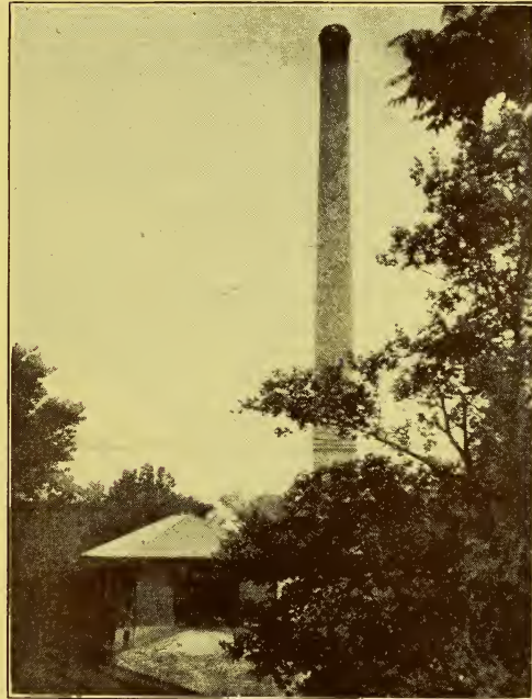
De-Carie Incinerator, formerly operated intermittently, now running every day. way repairs. The unsightly dumps are no more.
