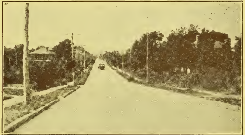
Graveled roadway laid by city forces on railless trolley route.
