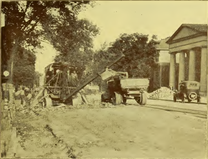
City equipment removing subgrade preparatory to repavement.
