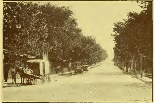
West Washington Street—Arterial roadway of concrete constructed in 1923.
